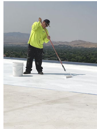
6) Apply 2nd topcoat layer.
