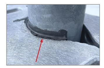
Zinc oxide can be easily removed using a mild acid such as cleaning vinegar. Lightly scrub the surfaces to be sealed using a nylon toothbrush dipped in cleaning vinegar. Rinse the surface with water and allow to dry before applying PIM Seal™ Caulk.
