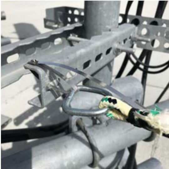
STEEL BANDING SECURING RF SAFETY ROPE
