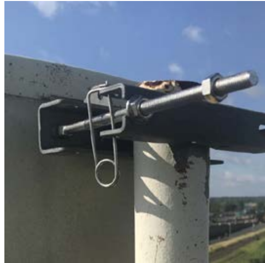
SPRING CLIP ON ANTENNA MOUNTING BRACKET
