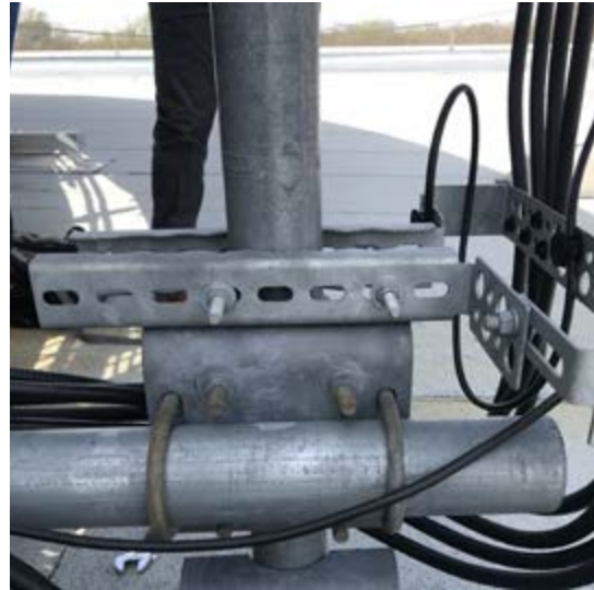
LOW PIM BRACKET CONTACTING SUPPORT BRACKET
