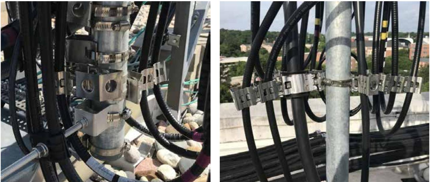
**Figure 8:** Traditional hardware used to secure the growing number of cables at cell sites
